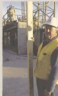
Far Left: New walls being constructed Image: Brendan Lee
