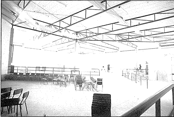
The new wing
