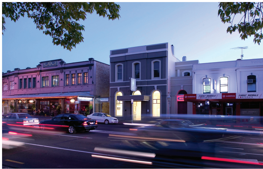
LIGHTS ON AND DOORS OPEN – OBJECTSPACE ON PONSONBY ROAD SHOWS ITS FACE TO THE EVENING TRAFFIC. ACKNOWLEDGEMENT: PATRICK REYNOLDS PHOTOGRAPHY
