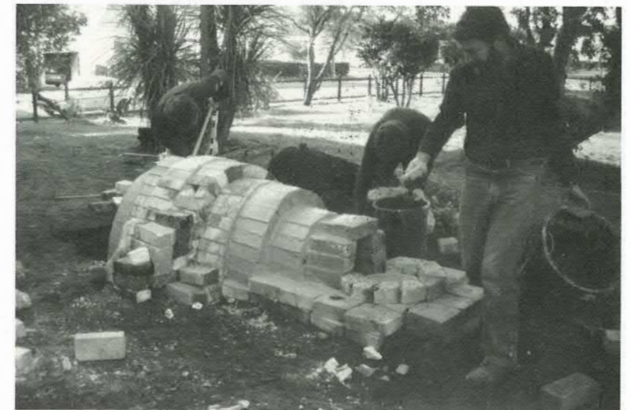
Chester and helpers build the body of the kiln.
