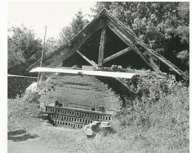
The rear of La Borne traditional kiln. There is no chimney — the flue exit is the lower half of the wall. During the final part of the firings a huge flame comes from this flue, covering the adjacent roadway and making it impossible to pass. After each firing the wall above the flue is dismantled to unload the pots and to pack the kiln again.
