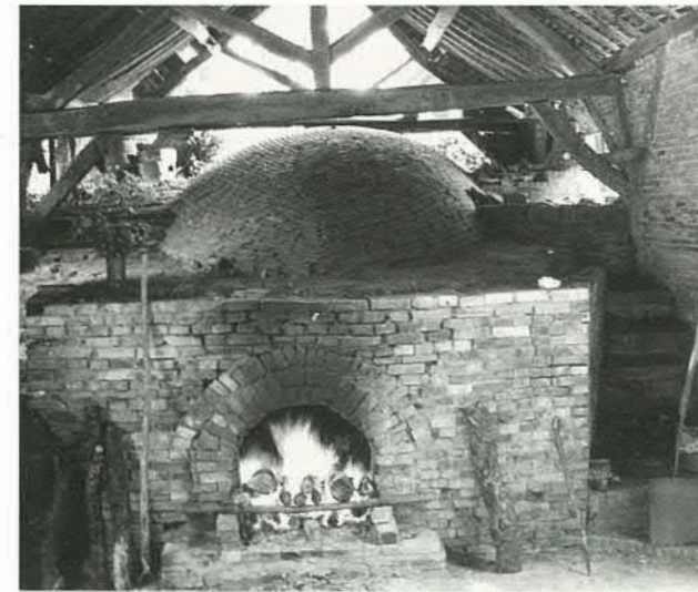
La Borne traditional wood-fired kiln. 25 cubic metres. This kiln was constructed at the end of 1800 and had been unused for many years until it was restored by the potters of La Borne. It was first fired again in 1977.
