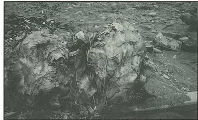
8. Eventual collapse of kiln walls
