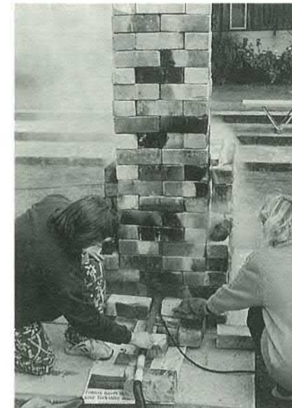
Firing on-site salt kiln
