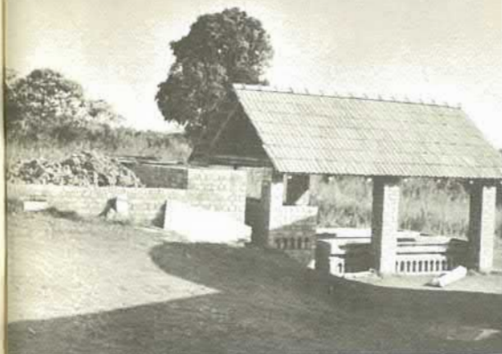
New clay preparing tanks
