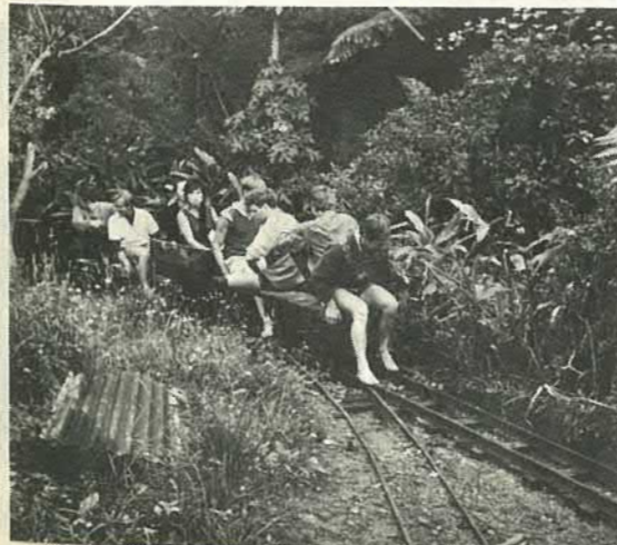
Driving Creek Railway.
