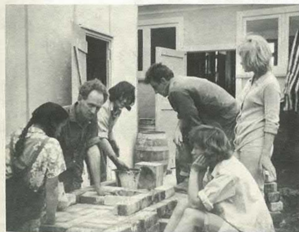
Peter Stichbury and students building a kiln at Ardmore
