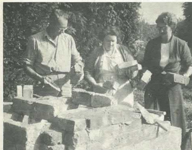
Building a kiln at Waimea College, Nelson 1959
