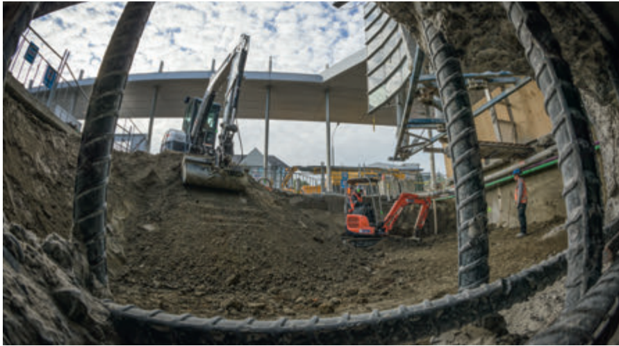
Excavations to enable repairs to the Gallery foundations
