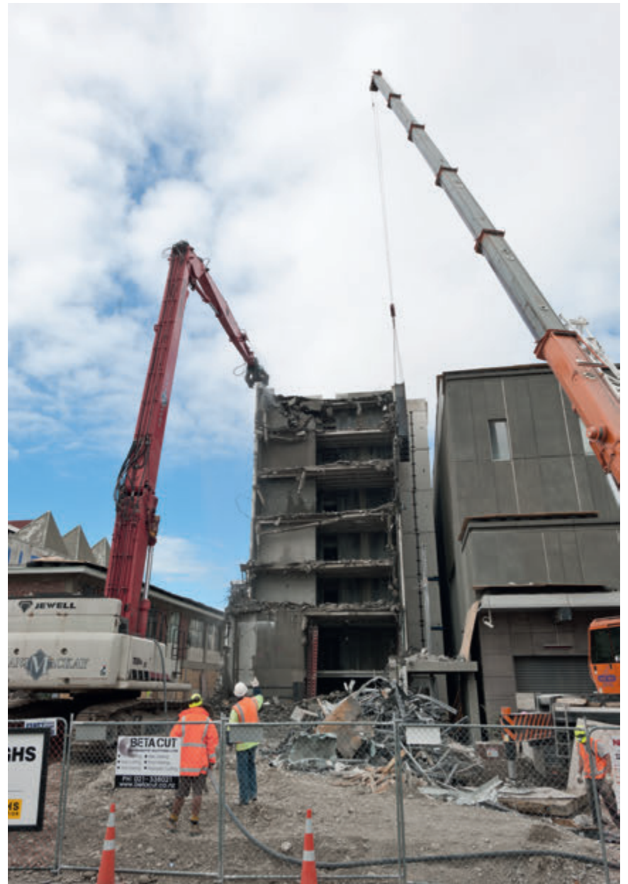
The Gallery Apartments next to the Gallery being demolished
